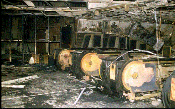
Kings Cross Underground Station fire (UK) 18/11/87 – 31 fatalities
