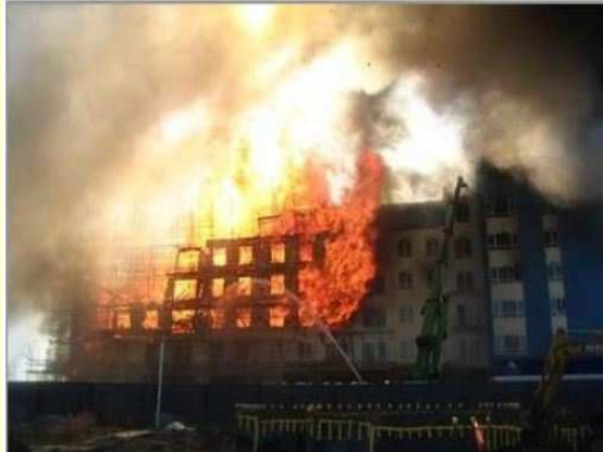
Collingdale 2006 Timber Frame Smoking
