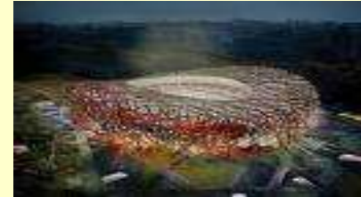
Beijing Olympic Stadium
