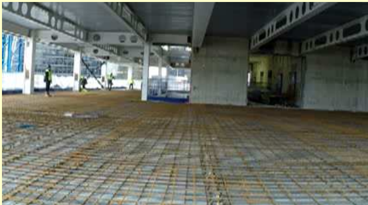
Person 1 walking across rebar
