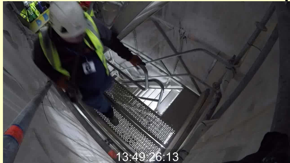
Layered stair down
